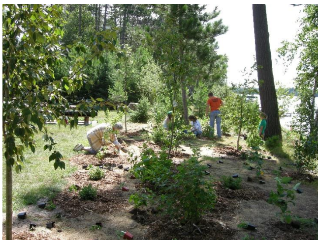
Shoreline buffer installation on a lake front property.
